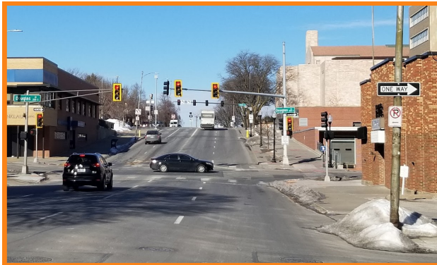
24th Street and Douglas Street Retroreflective backplates on signal heads
