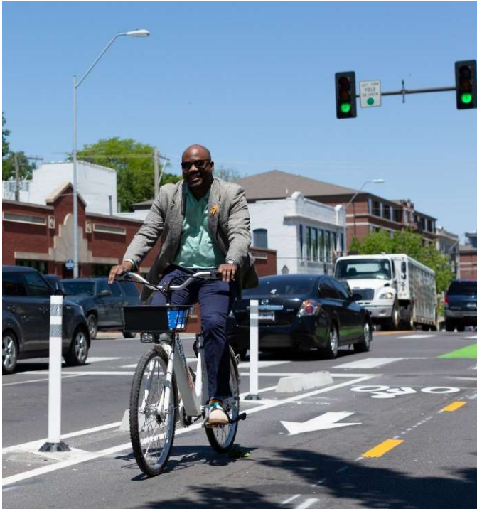
Quick Build Protected Cycle Track
