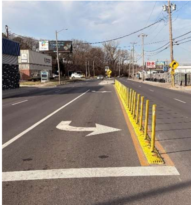
Quick Build Lane Separators
