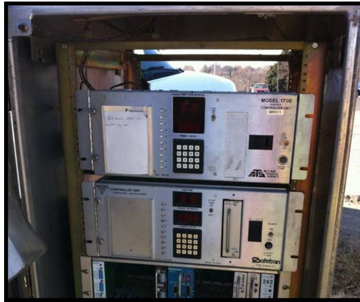
FIGURE 2 – TYPE 170E LOCAL AND MASTER CONTROLLERS
