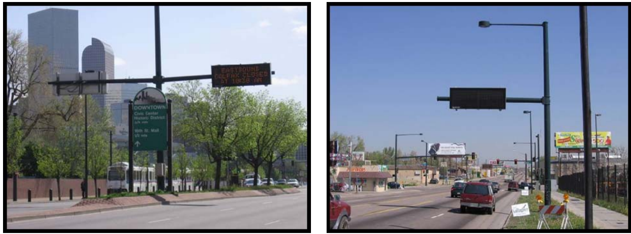
FIGURE 16 – EXAMPLES OF SINGLE- AND DUAL-SIGN CANTILEVER DMS INSTALLATIONS
