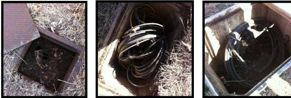
FIGURE 6 – TYPICAL VARIED PULL BOXES AND FIBER VAULTS
