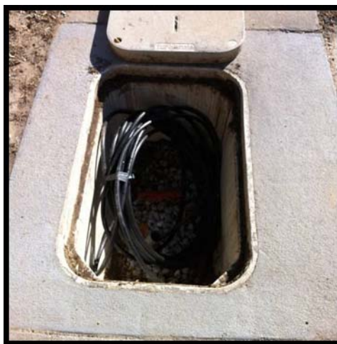
FIGURE 8 – TYPICAL UNITE PRIVATE NETWORKS FIBER VAULT
